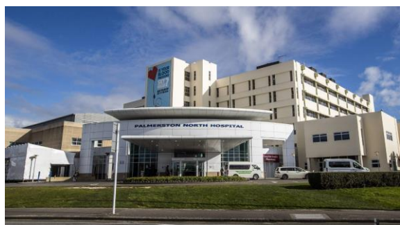
Palmerston North Hospital
